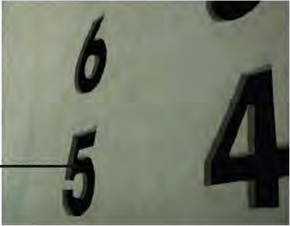
Example of precast concrete treatment for sign
